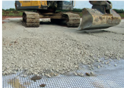
Construction of roads with unbound surface courses
