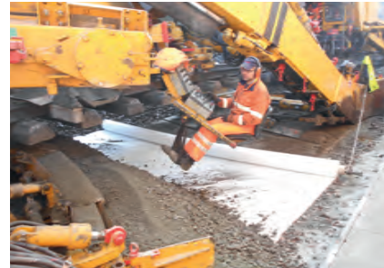
Installation of reinforced base courses in railway engineering
