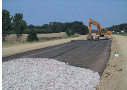
Installation of reinforced base courses for highways
