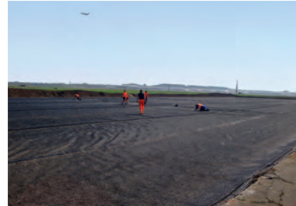
Installation of base courses in airport engineering and runway shoulders
